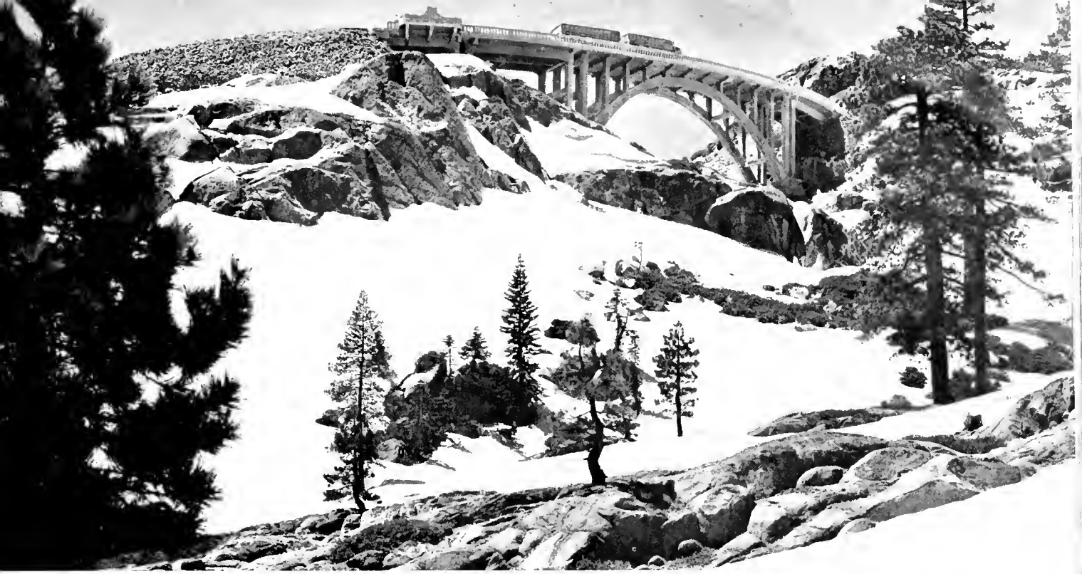
A "dry land" bridge on a summit used in place of a more expensive fill with retaining walls
